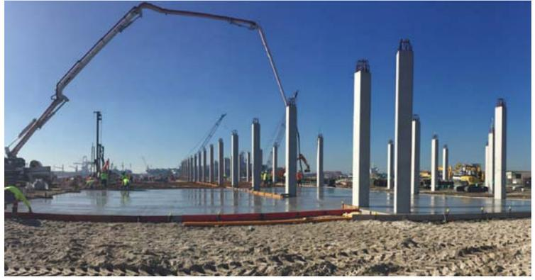
**CONSTRUCTION** work on Brisbane's new International Cruise Terminal is proceeding apace, with almost all of its 107 wharf piles installed and major civil works including concrete pours and the base of the new terminal building in progress.
