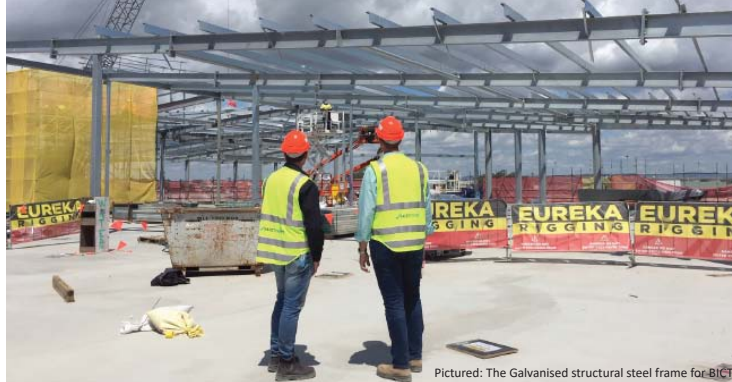
Pictured: The Galvanised structural steel frame for BICT.
